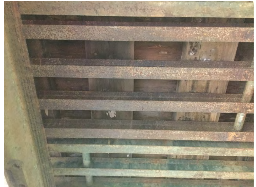
Deck from underneath
