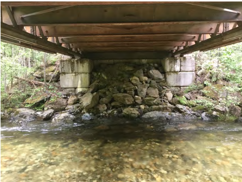
Right Bank Abutment when facing downstream
