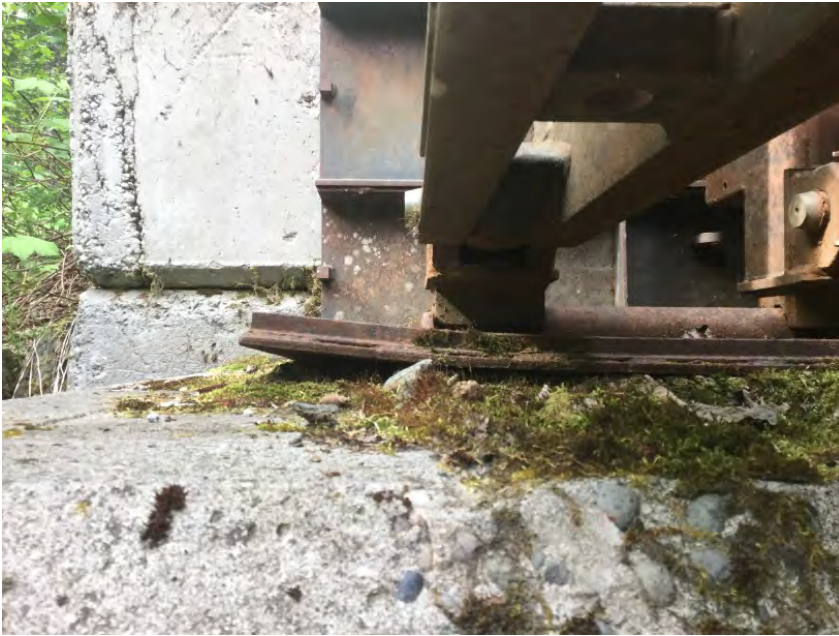
Upstream left bank bearing plate
