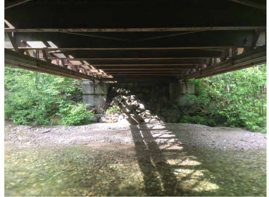
Left Bank Abutment when facing downstream
